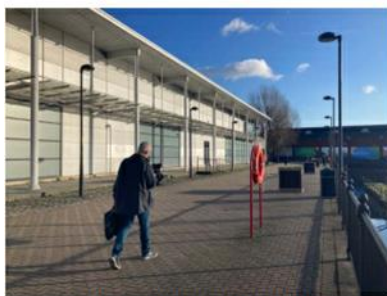
EXISTING BUILDING FROM DOCK EDGE
