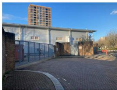
EXISTING SERVICING ACCESS
