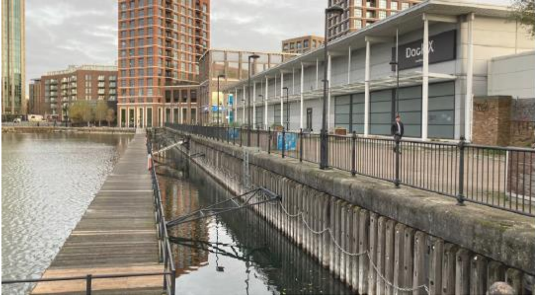
Image above: Floating fishing pontoon located along the eastern edge of the dock
